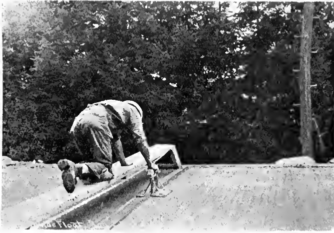
Fig. 4.—Divided float in use at expansion joint.
